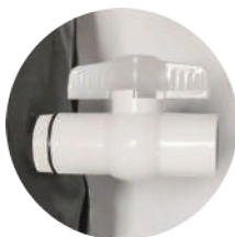
Ensure drain valve is closed.
